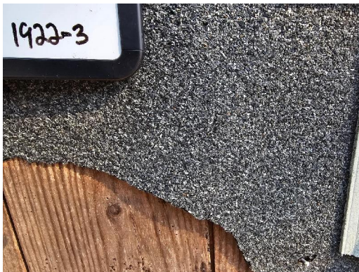
1922-3 Asphalt House Wrap Typical Exterior Walls
