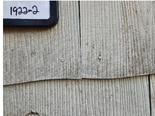
1922-2 Transite Siding/Gray (13% Chrysotile) Typical Exterior Walls
