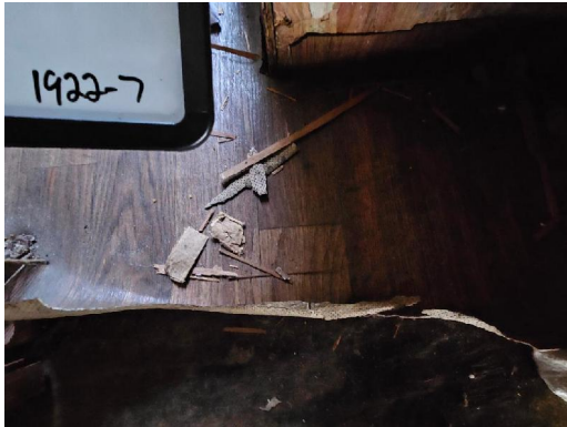
1922-7 Rolled Flooring Interior Bathroom
